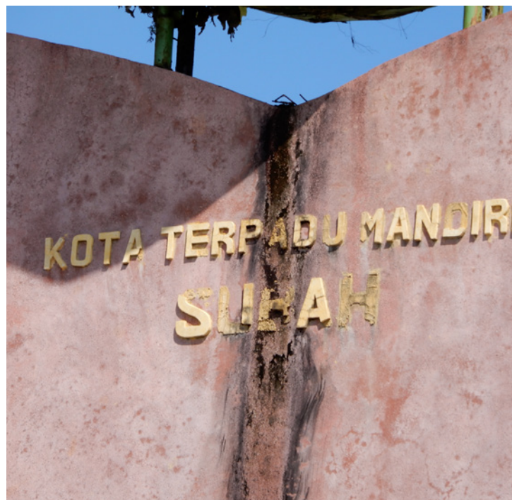
KTM Subah now symbolises decay and neglect
