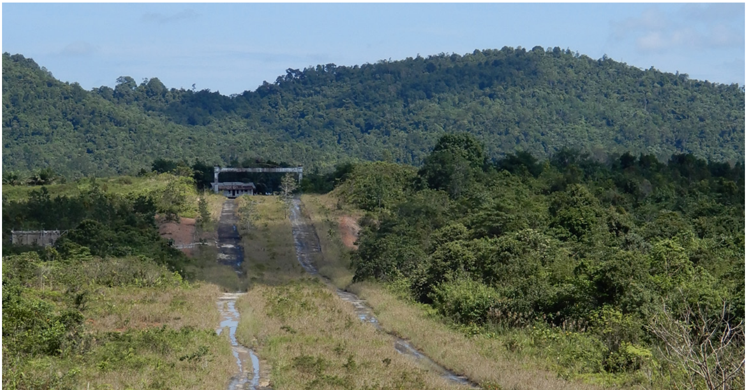
Roads are collapsing back into mud and ruin
