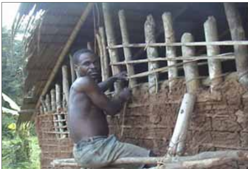
House building © CED
