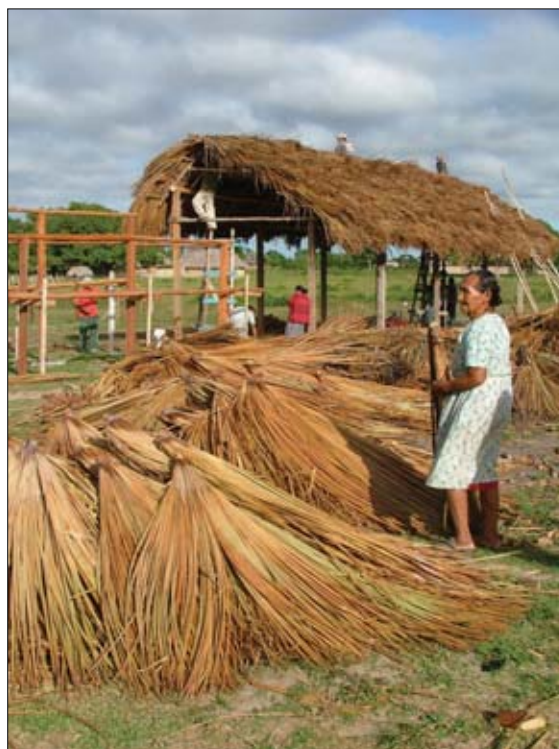
Dyuwuza anaba – Ité palm leaves being used to thatch village sports pavilion, Aishara Ton, 02/05
